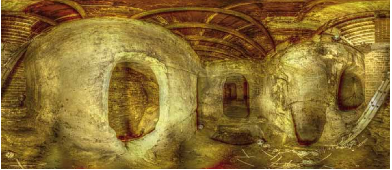
The medieval malting below Birkin's lace warehouse. 360-degree panoramic image, showing (left to right) the malt kiln, germination floor, well and cistern. Note the carved crosses and the pulley-beam slot above the well.
